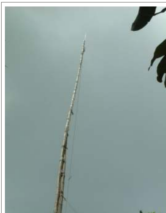
This is not a joke! This station works. At Y-Echo FM, Kataka, Liberia, the antenna mast is bamboo and the antenna is a kitchen knife! Every rural community in Nigeria can do that!
