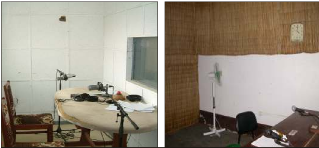
Right: Radio Kasumai achieved soundproofing using mats; another station uses professional-standard soundproofing. Always go for what your community can afford.
